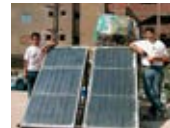
▲ Pipes inside our solar panels heat the water.
