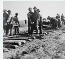
▲ Workers lay new track for the railroad.
