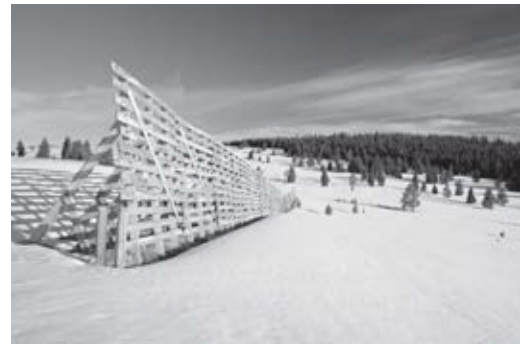
▲ Snow fences trap blowing snow.
